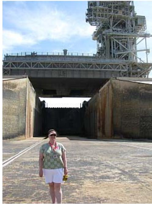
Kat Sarbell at the opening to the flame trench. This was our second stop at the pad. The blast deflector is visible in the trench under the Mobile Launch Platform. It deflects the SRB exhaust out this way and the main engine exhaust out the other way. The floor and walls of the trench are covered with refractory bricks. The bricks were blackened and really pitted. You didn't want to be here during a launch!!
