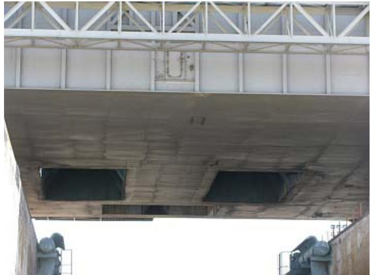
The bottom of the Mobile Launch Platform with the two openings that the SRBs fired through in the foreground and the opening for the Shuttle Main Engines in the back. In the lower left and lower right are nozzles that blast water from the large water tank into the flame trench during a launch.
